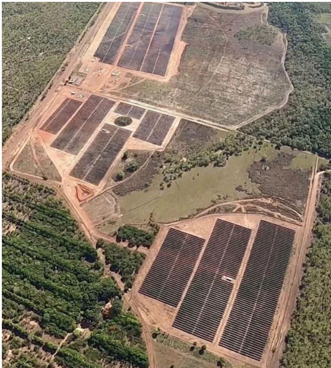
Figure 7 Solar farms at Batchelor (Batchelor 1 and Batchelor 2) adjacent to the Winchester project
