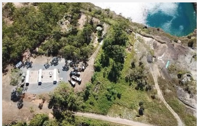
Image 1: Mt Chalmers Site Works Progress, January 2022.
