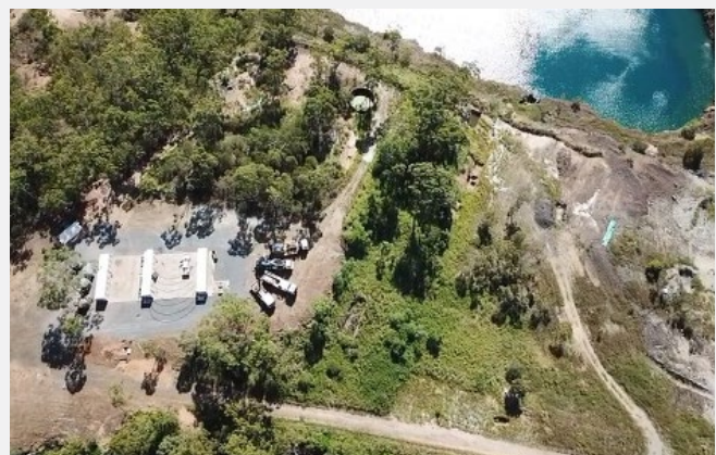
Image 1: Mt Chalmers Site Works Progress, January 2022.
