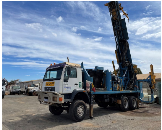
Image 2: RC Drill Rig Delivered to Mt Chalmers Site.
