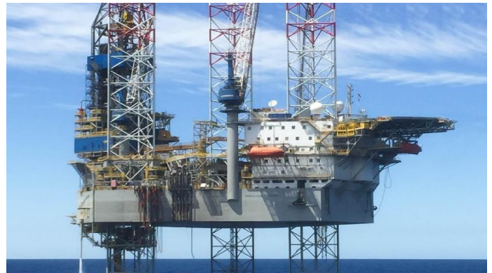
Photo of the Noble Tom Prosser drilling rig
