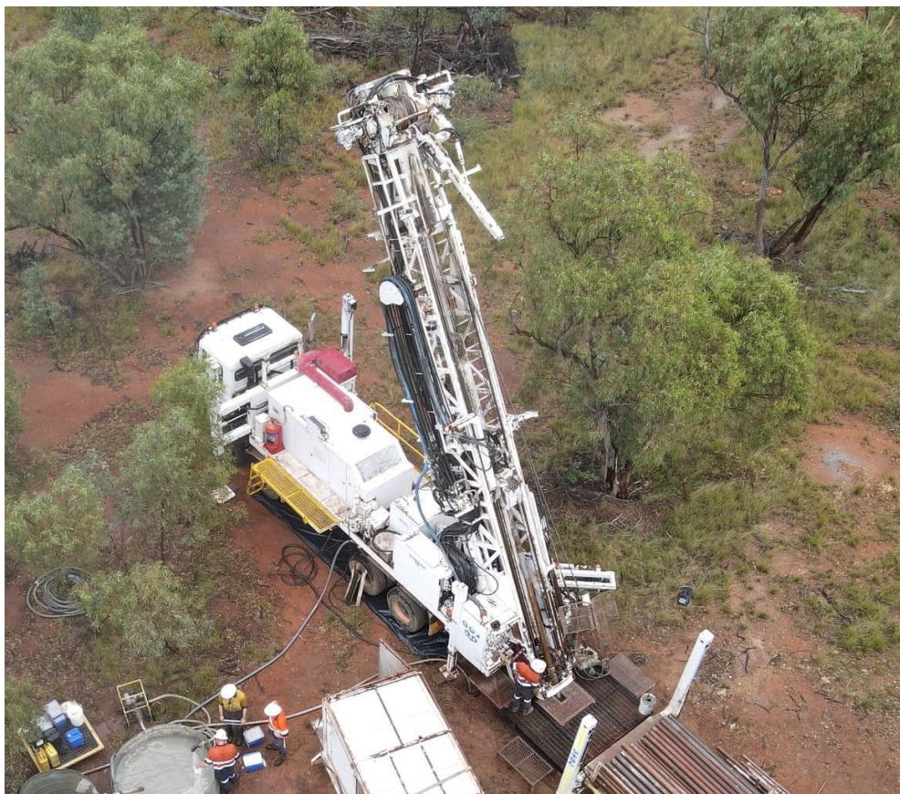
Figure 2. Drilling underway at Pearse North
