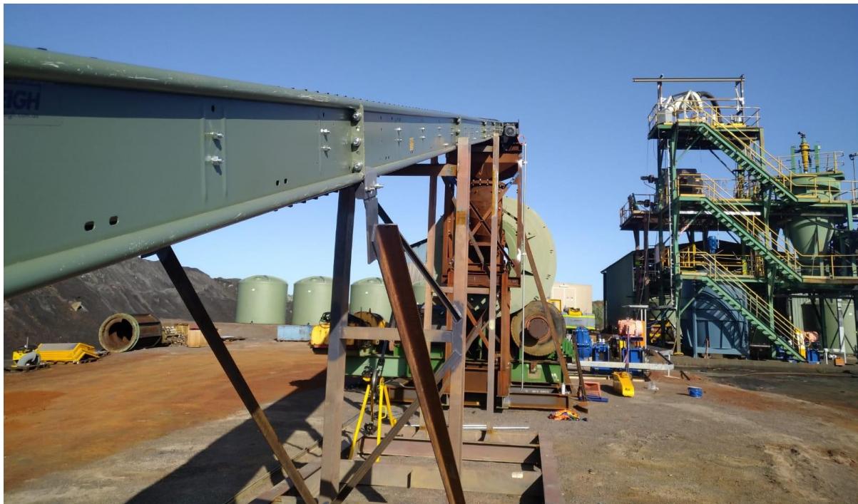
Process water tanks, mixing tanks, cyclone and magnetic separator tower in the background
