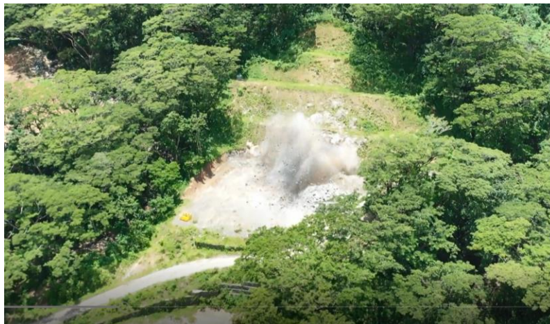
Photo 2: blasting for development of underground access no.2
