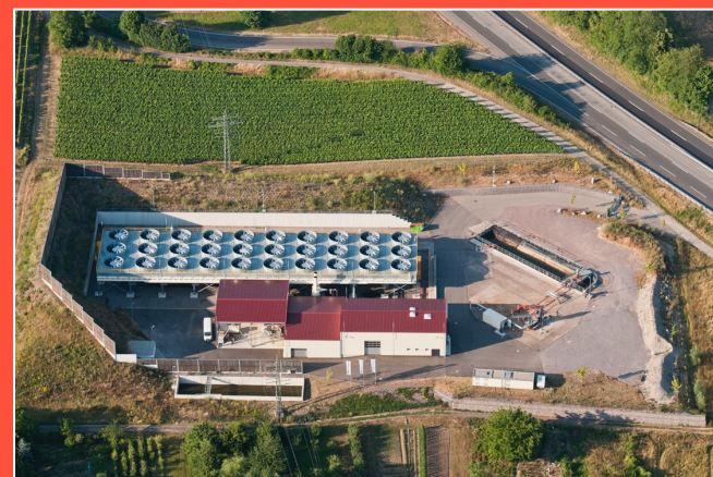
Geothermal Plant Insheim (A1)
