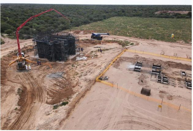
• Primary Crusher vault first lift reinforcing above.
