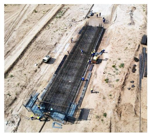
• Base slab reinforcing installed and ready to pour.
