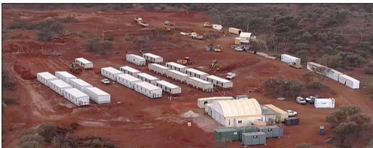
Figure 3: Camp Installation has commenced with the first 80 rooms landed and dry mess installed.
