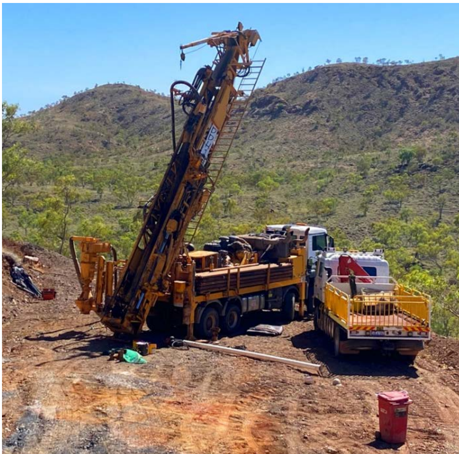
Figure 5. Drill Rig on site at K-142
