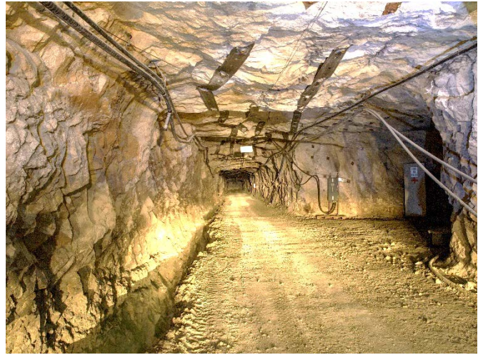
Photo 2 – Underground intersection showing good ground conditions, and existing air and water services
