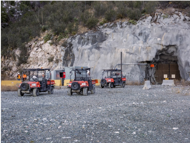
Photo 7 – Portal to Underground. Note rehabilitated portal entrance with shotcrete support
