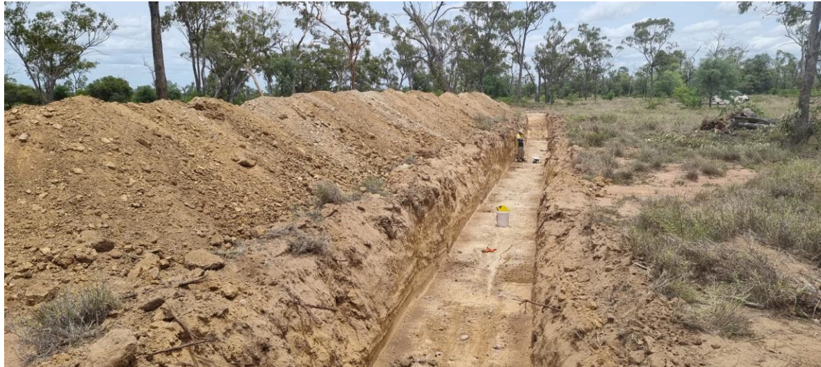
Image 1: Operations at the first trench of the phase two trenching program
