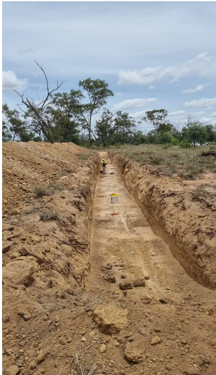
Image 2: Operations at the first trench of the phase two trenching program
