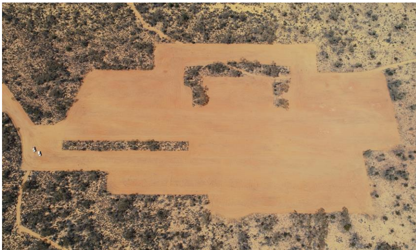
Topsoil and Subsoil Removal at the Accommodation Village Location looking south (24 November 2021)
