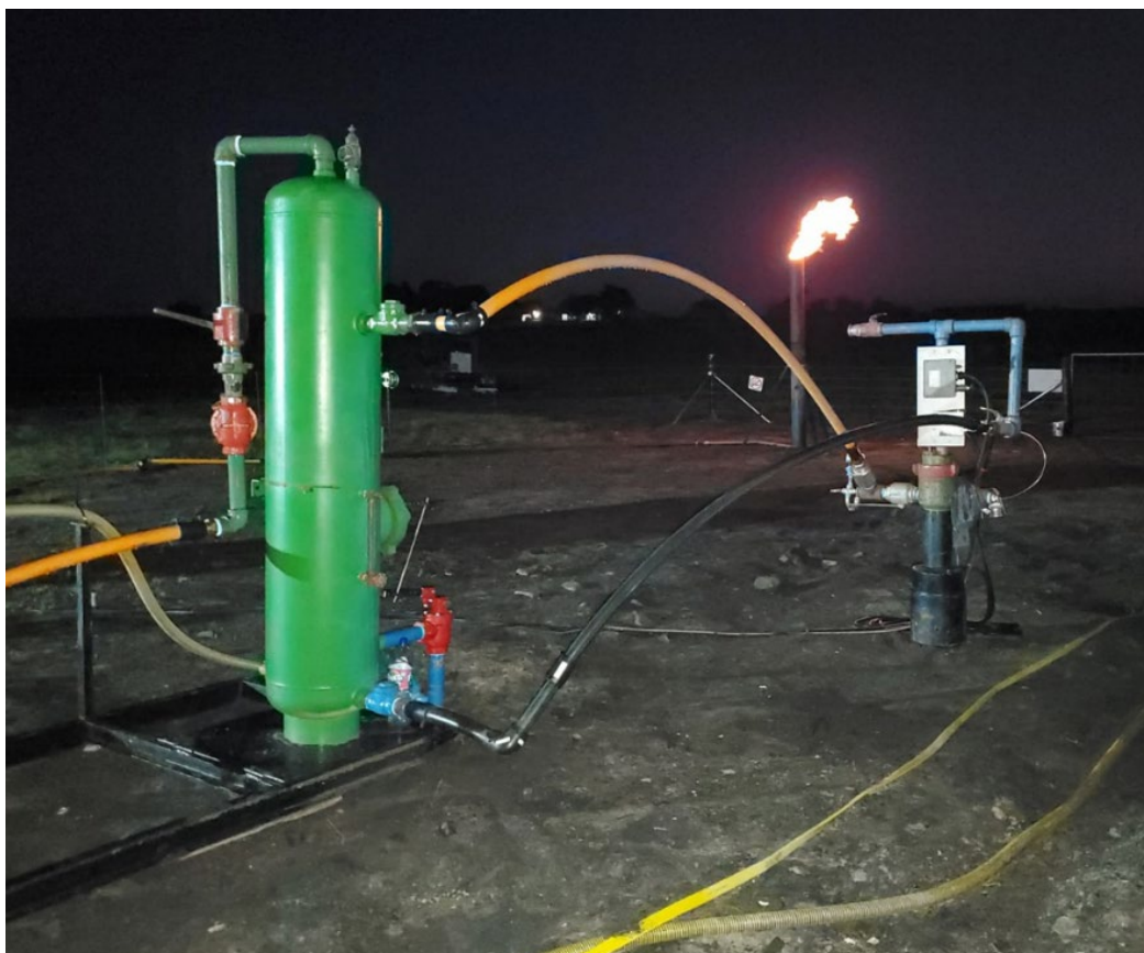
Figure 2: Blowing down pressure build up on Korhaan-5 prior to pulling the pump string on 11 Feb 2022
