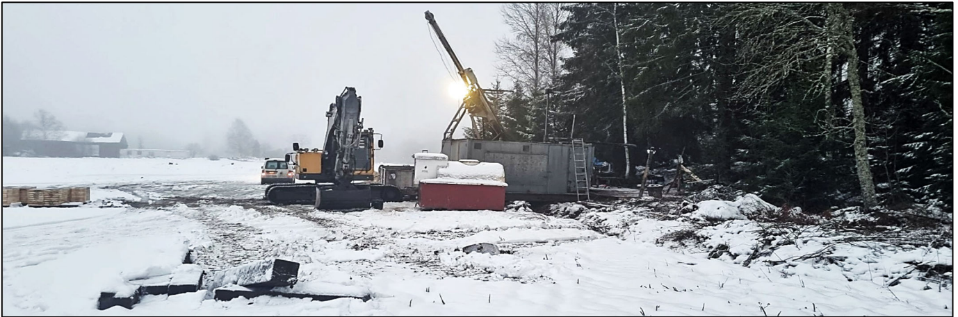
Figure 3: Drilling during the winter months at Granmuren.
