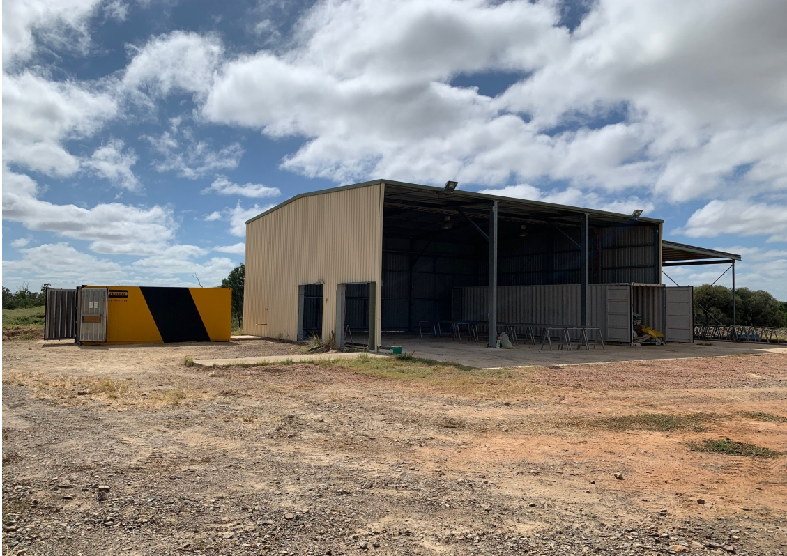
Figure 6: Original mechanical workshop now being re-purposed as dedicated core logging and processing facility. The yellow container is an airconditioned core cutting room that will house a new Corewise™ automatic core saw.
