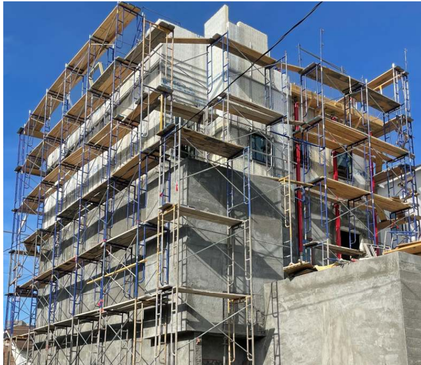
Figure 1. 4-storey SCIP residential home in Houston under construction and including EdenCrete ®
