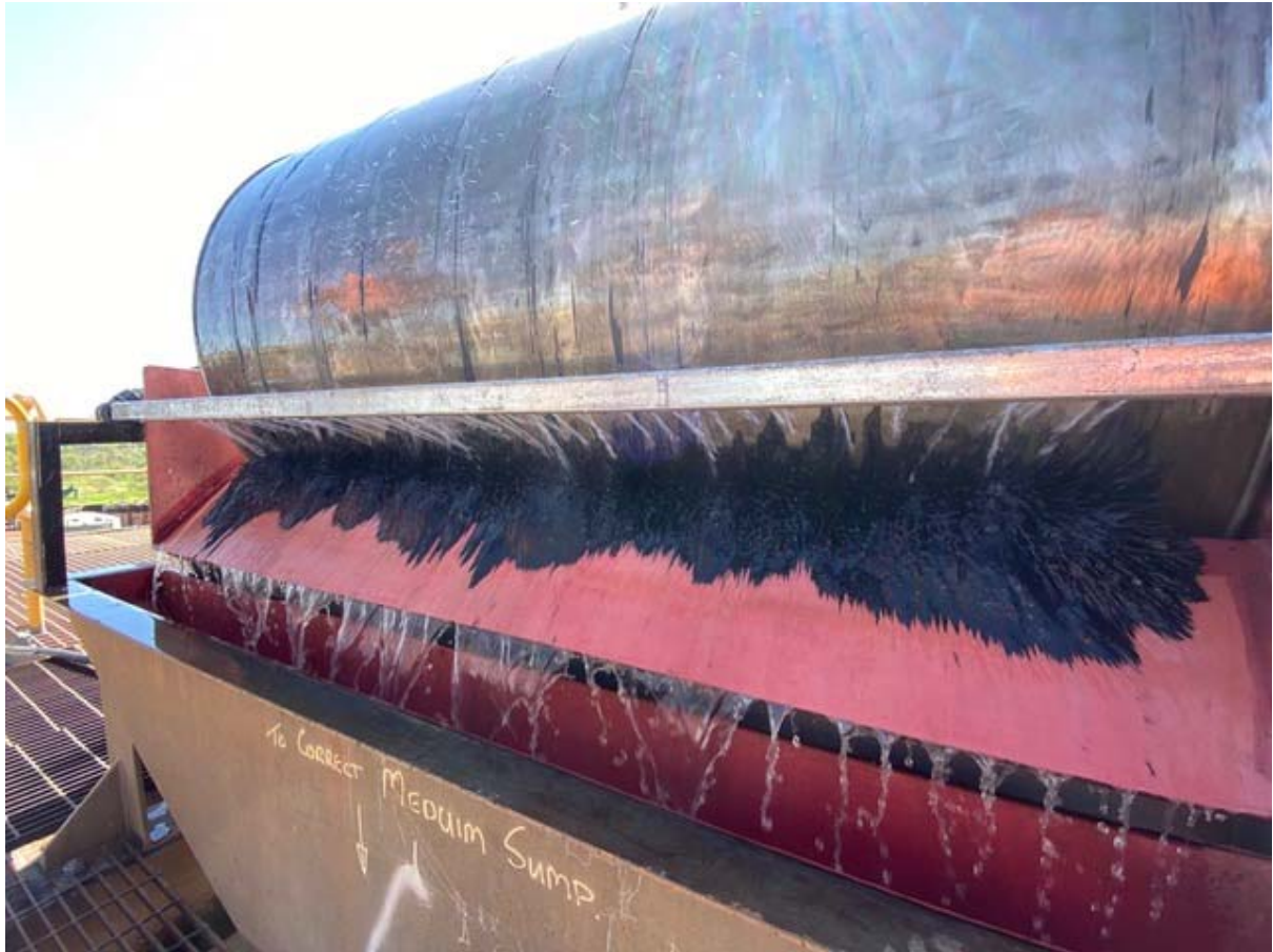
First magnetite product produced out of commissioned magnetic separators.
