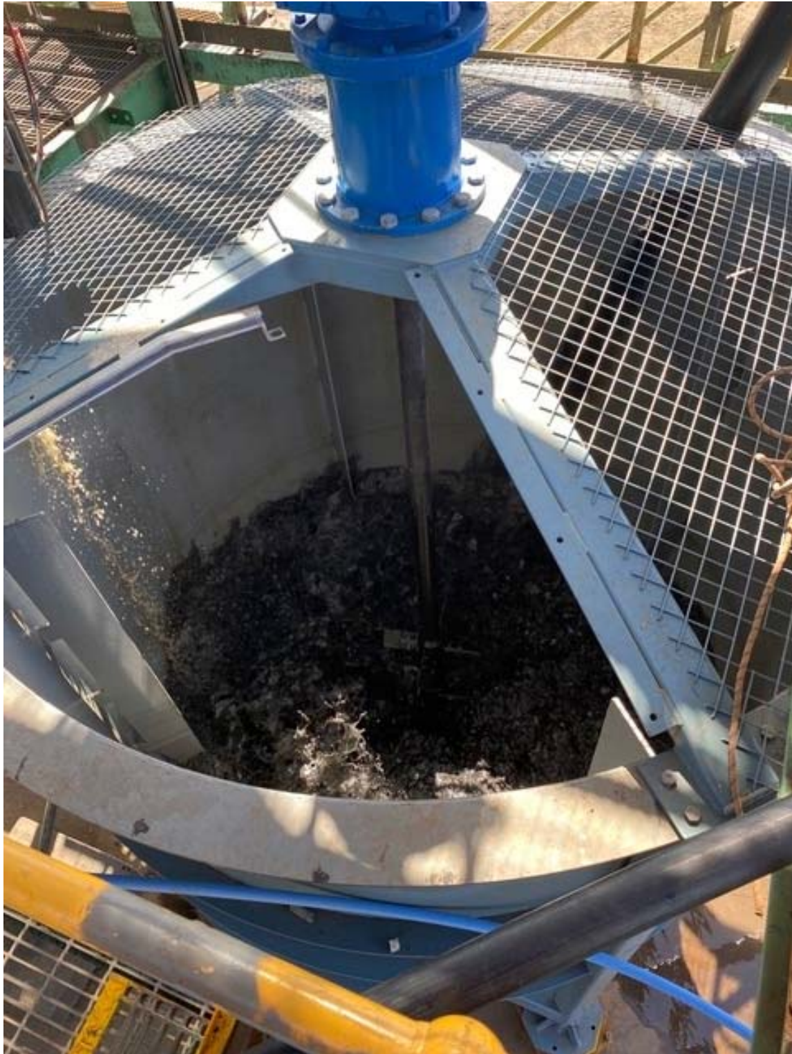
Magnetite rich slurry in commissioned primary mixing tank
