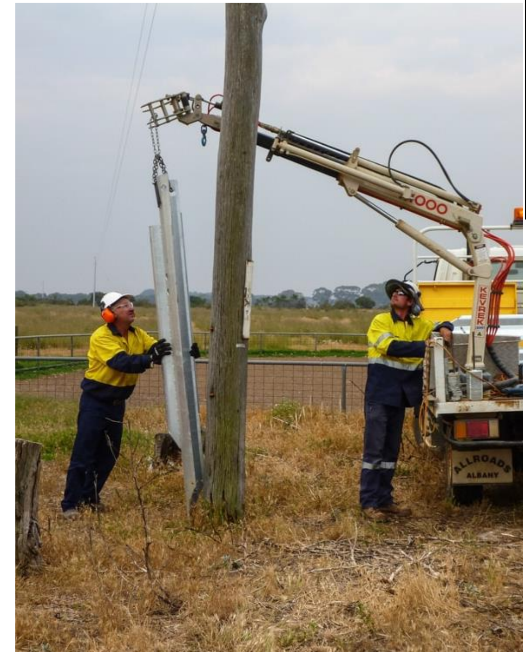
Installation of wooden pole reinforcement
