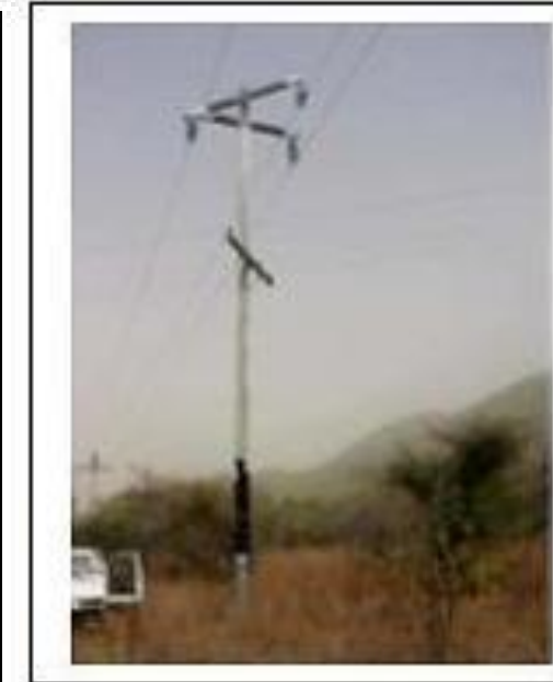
↑ Ergon Energy photo taken in Queensland, Australia showing the height at which the power pole was burnt, when a bush fire went through the area. A Powerbeam, reinstated prior to the fire, is seen at the base of the pole
