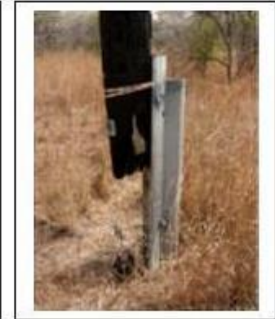
↑ Ergon Energy photo (side view of photo ←) showing how the entire base of the power pole was burnt, then washed away in the aftermath of a flood
