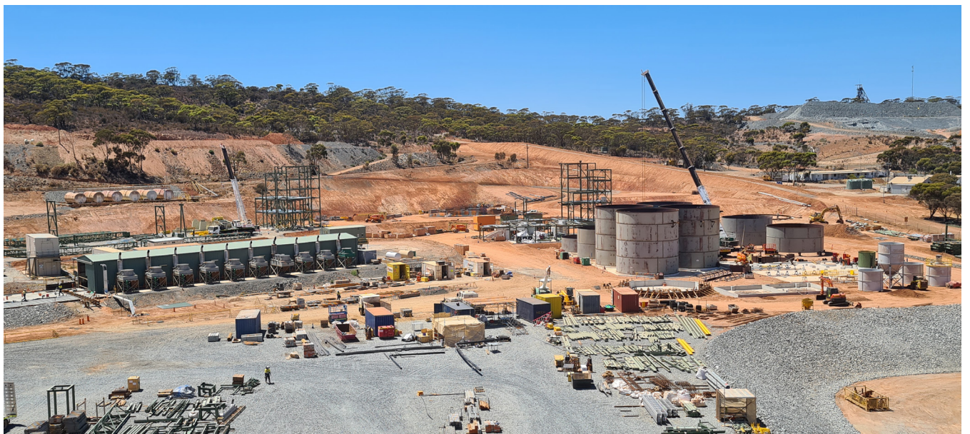
Construction activities progressing as planned.
