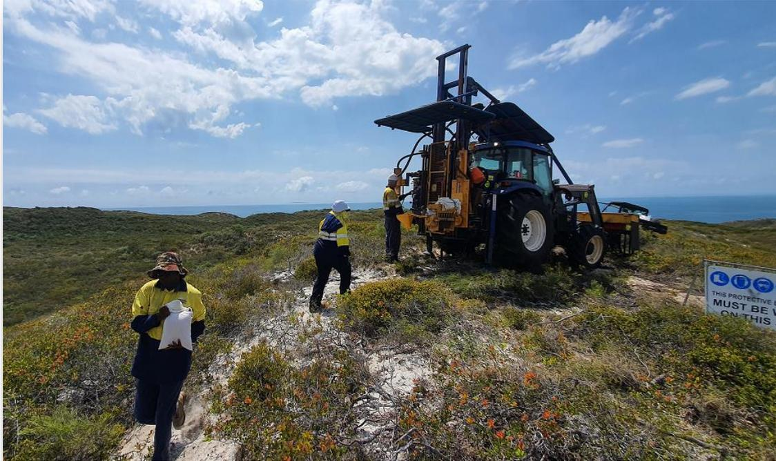
**Figure 10: Si1 South vacuum drilling in progress**
