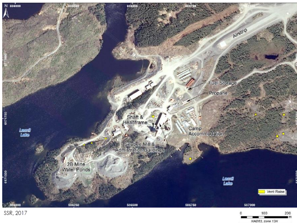
Figure 18.2 Seabee Gold Operation Mill Site Infrastructure
