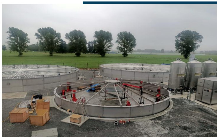
Image 1: Ecogas tanks construction
