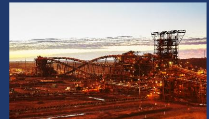
Christmas Creek Hydrogen Refuelling Station ($7m)
