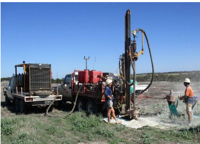
Fig 1: Drilling on Kelly Tank 26 Feb 2022
