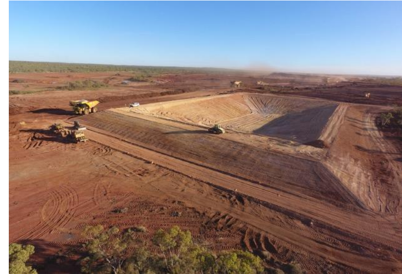
50 megalitre water storage dam ready for lining.
