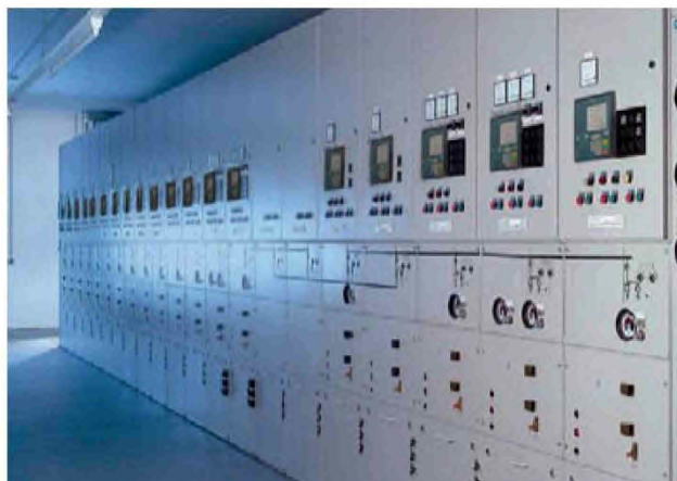
Figure 15 - Typical 33kV GIS collector switchboard (Siemens 8DA10)
