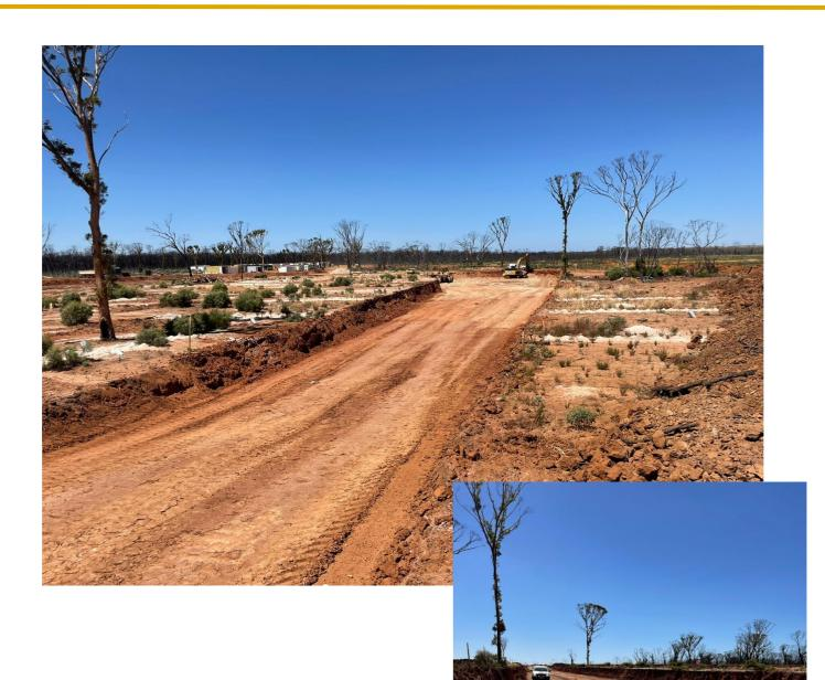
Figure 4: Views of Initial Ramp into Pit.
