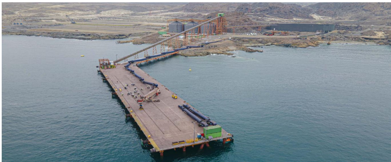
Concentrate loading facilities at Las Losas port, adjacent to Hot Chili's Costa Fuego copper-gold project, Chile
