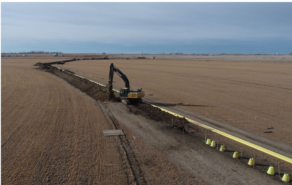
Installation of 6” Pipeline at Brooks
