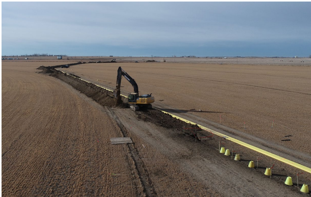
Installation of 6” Pipeline at Brooks
