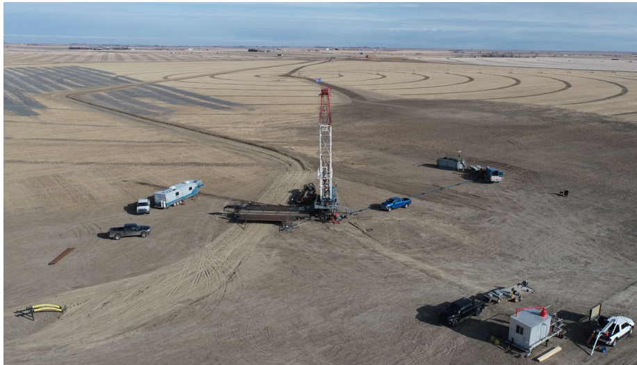
Service rig performing completion activities on Gemini well at Brooks
