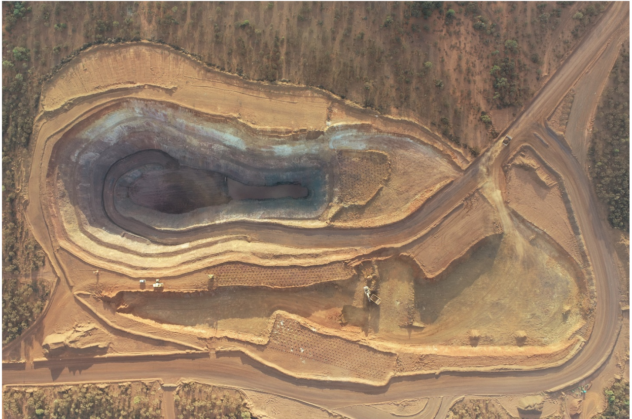
Figure 1: Aerial view of the high-grade C4 iron ore pit as of the 1 st March 2022 showing the Stage 2 cut back taking shape
