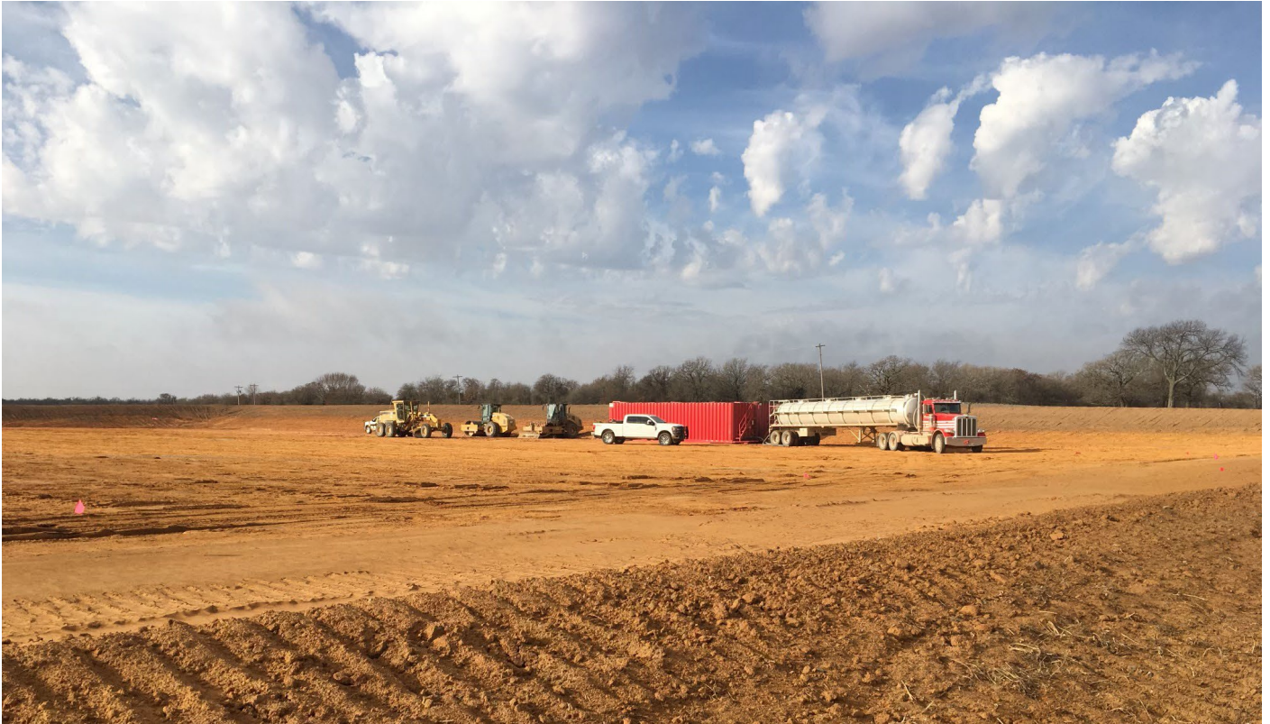
Figure 1. Flames DSU multi-well all-weather pad under construction in Carter County, Oklahoma
