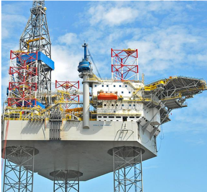
Dorado discovered in 2018 & appraised in 2019. Photo of Noble Tom Prosser drilling rig.
