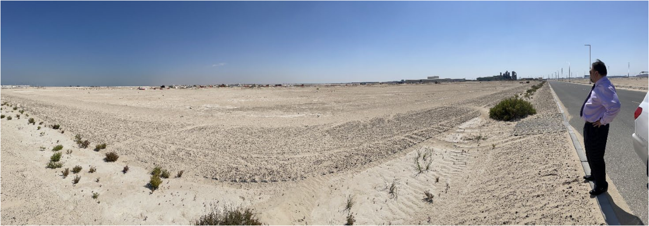
Faysal Khan, Commercial Manager UAE inspects the Phase 1 chemical plant site looking eastward
