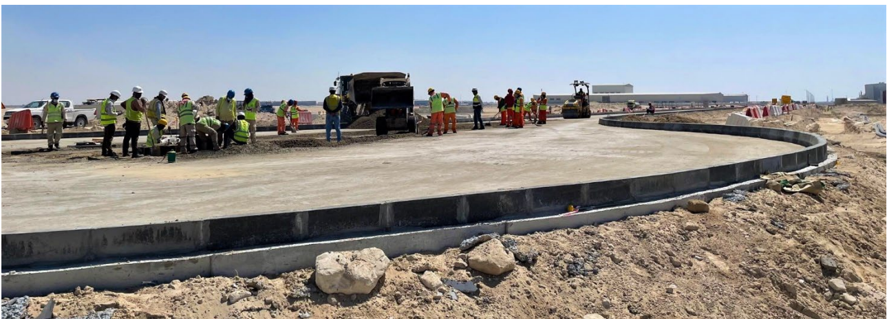
Access road construction works were well advanced, 6 March 2022
