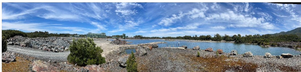
Figure 9. Avebury Tailings Storage Facility and Plant (Source: MYL)
