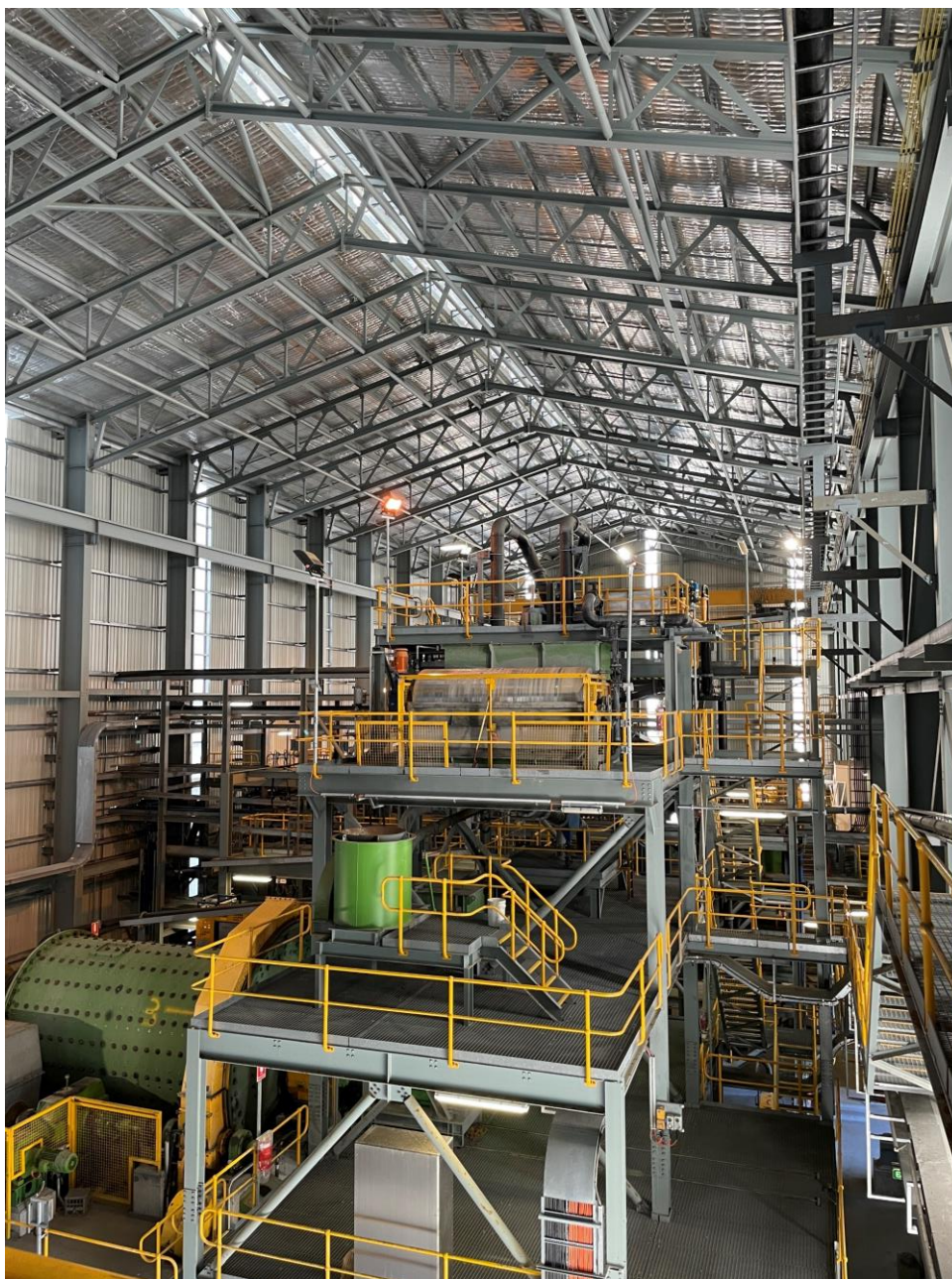
Figure 7. Avebury Processing Infrastructure Shed (Source: MYL)
