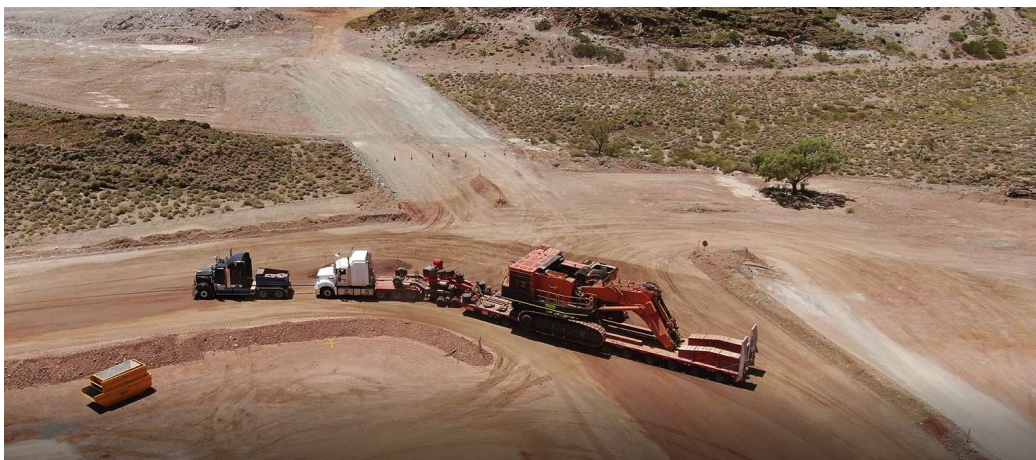
Figure 8: 200t excavator mobilised to Warrawoona
