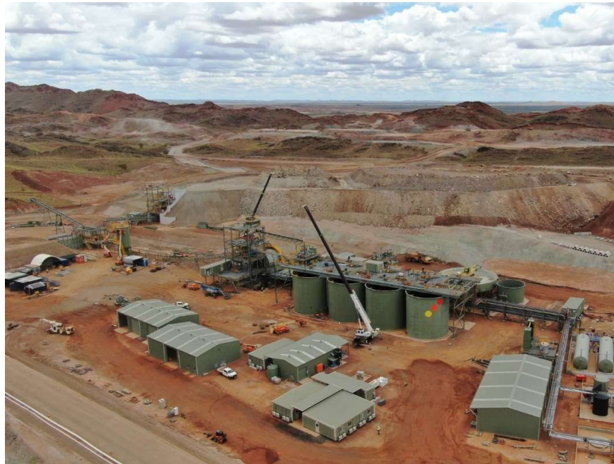
Figure 3: Process Plant Construction – Site View
