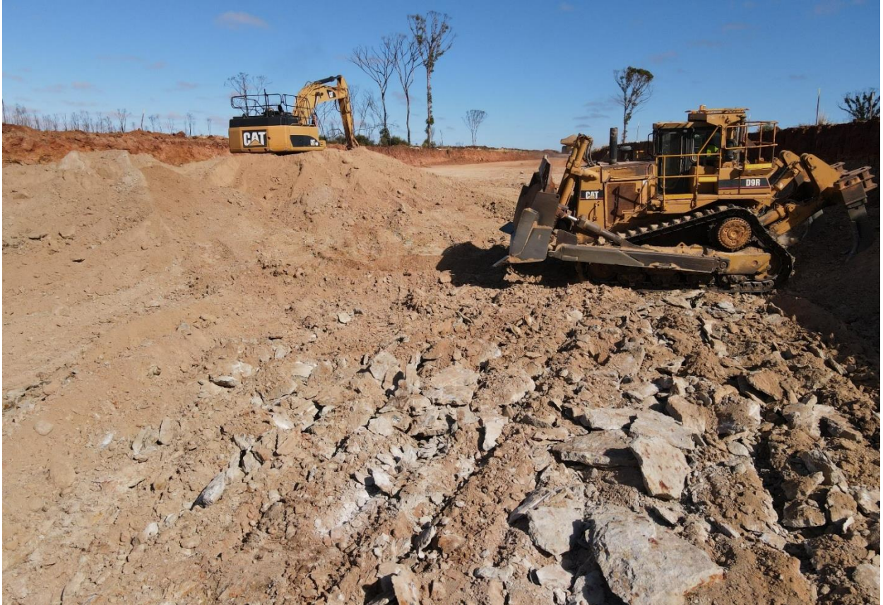
Figure 3 & 4: Bulldozer and excavator in pit.
