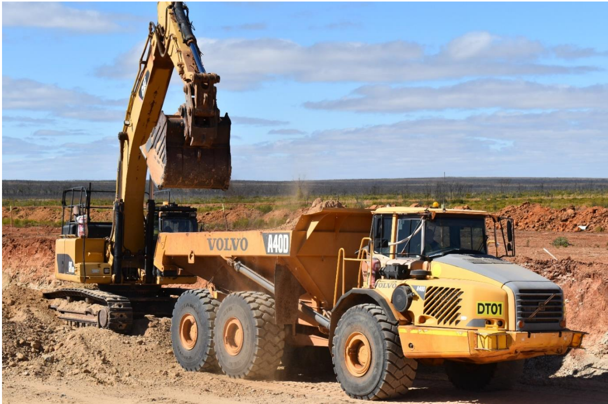
Figure 5 & 6: Excavator loading dump truck & Dump truck going to waste pad
