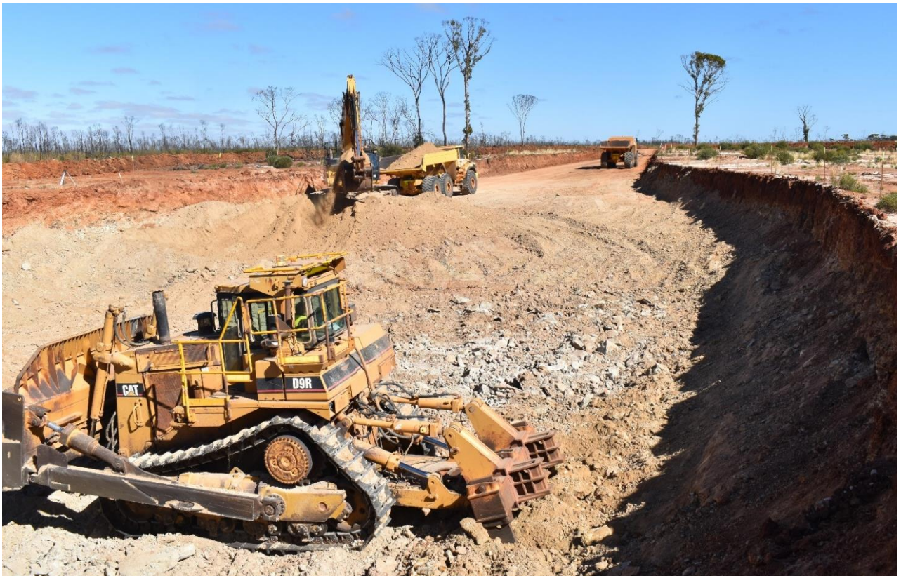
Figure 2: Bulldozer ripping pit floor
