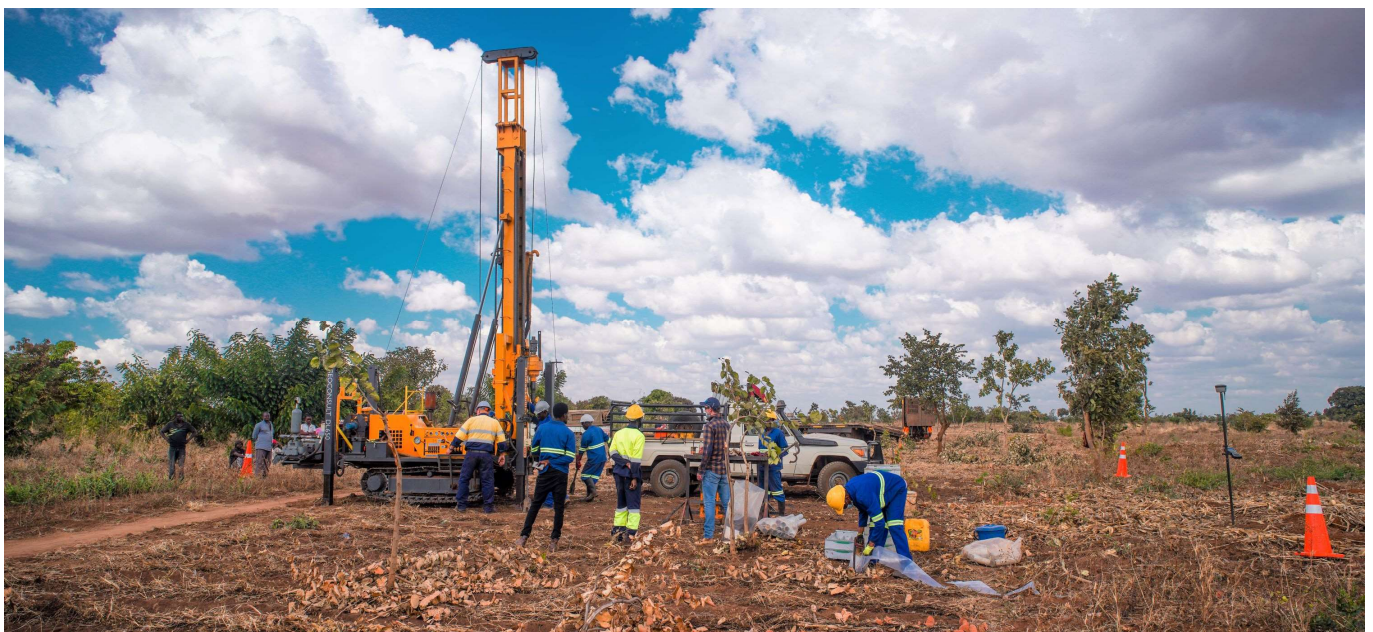
Figure 2: DL650 push-tube core drilling rig in operation at Kasiya-Nsaru
