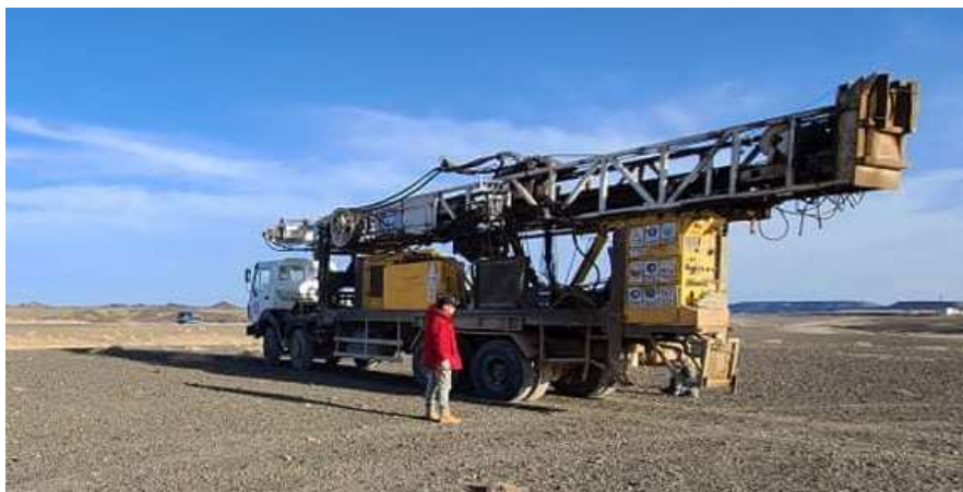
Drill Rig mobilised to site
