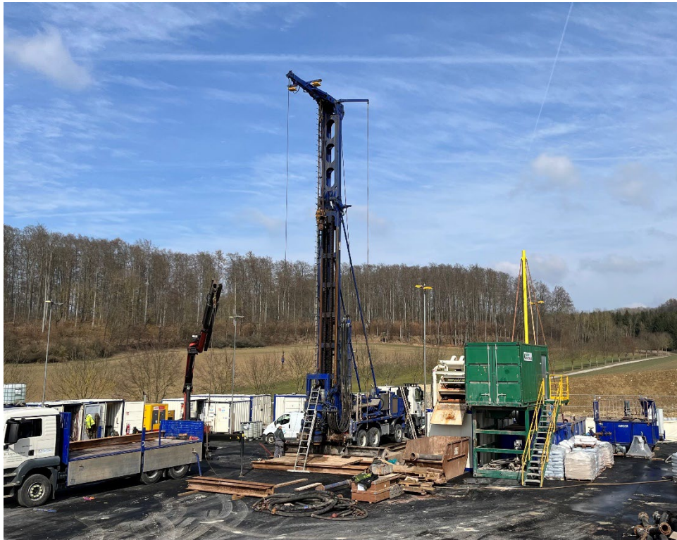
OHM-02 drill site with drill rig in centre
