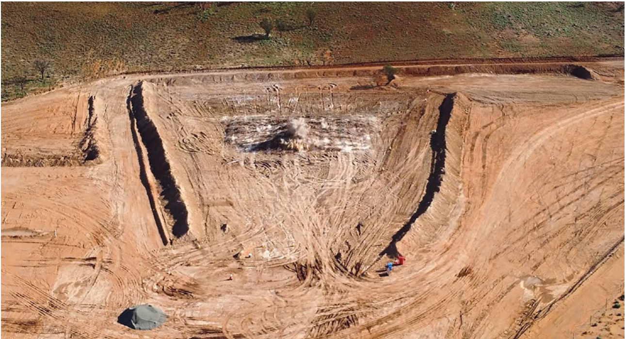
Figure 1 – Initial blast to advance excavation of the Pyrite Hill box cut.
