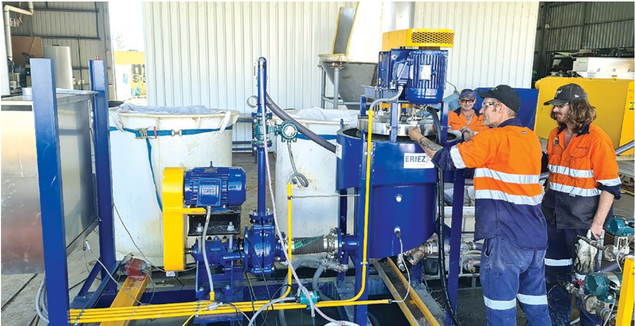
Figure 3 – Commissioning of the float cell
