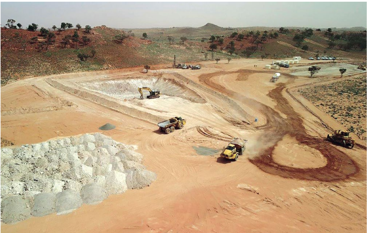
Figure 2 – Load and haul activities at the Pyrite Hill box cut.
