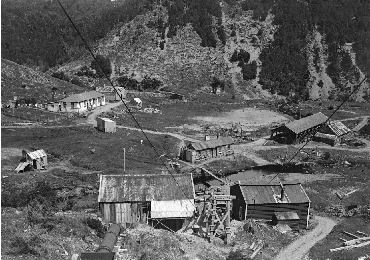
Figure 4. A photo of the Historic Big River battery (foreground) and cyanide tanks (in the shed middle RHS).
