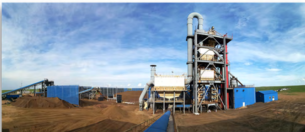
Figure 11: “Plug & Play” Dry Magnetic Beneficiation Plant
