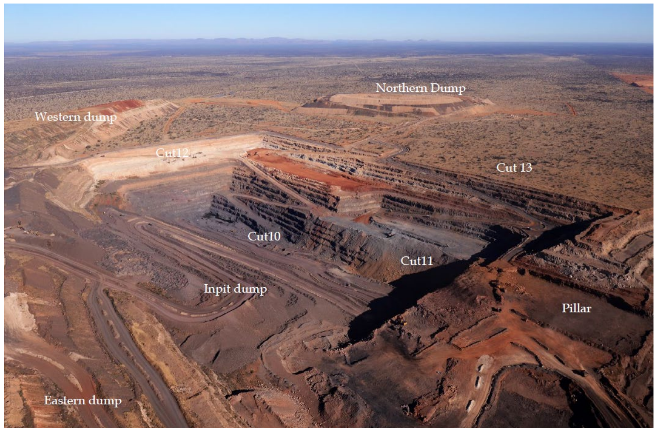
Figure 1: Overview of Tshipi pit
