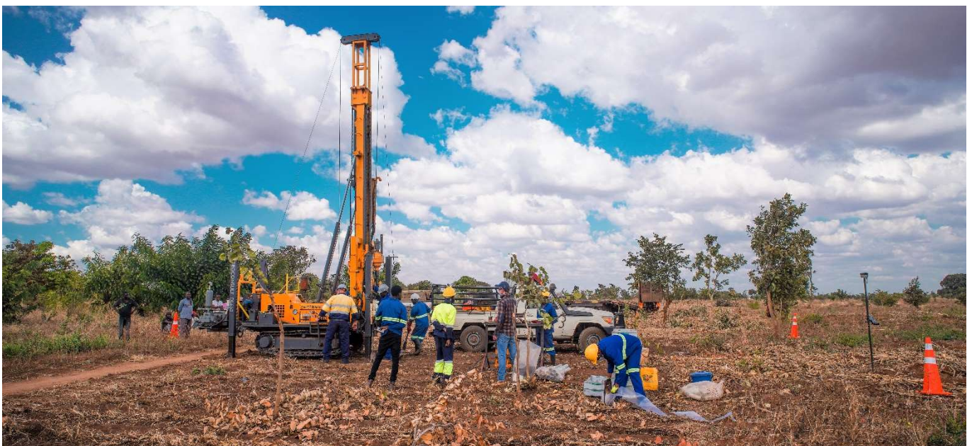
Figure 13: Core drilling in action at Kasiya
