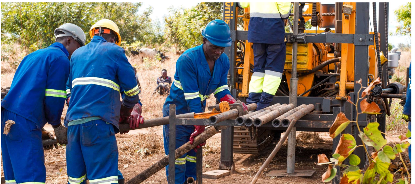
Figure 5: Core drilling at Kasiya
