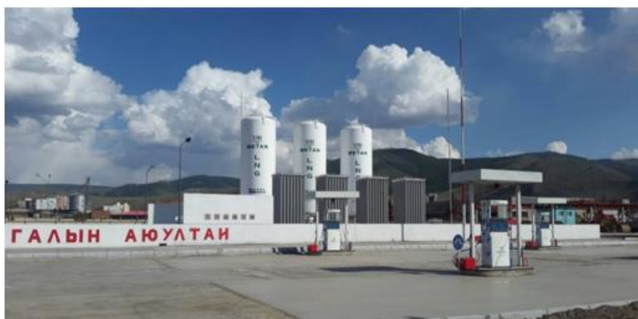
View of commissioned L-CNG fuelling station
