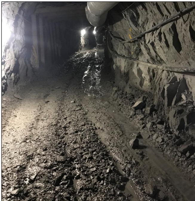
Figure 2 - In Progress Development Drive
