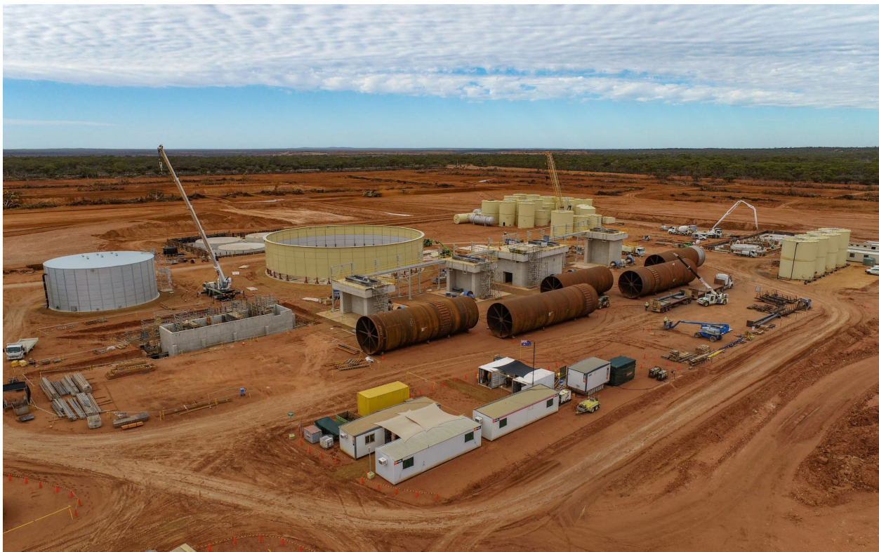
Aerial view of Kalgoorlie construction works, March 2022
