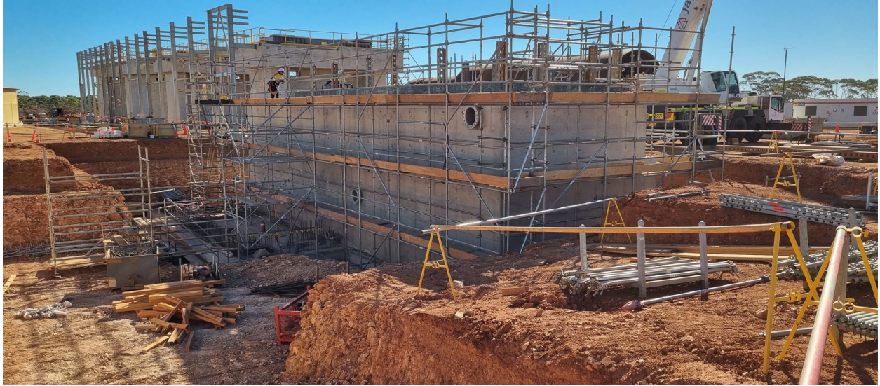
Primary leach area with kiln piers in background
